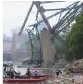
The collapse of the I35w in August last year focused US attention on infrastructure
